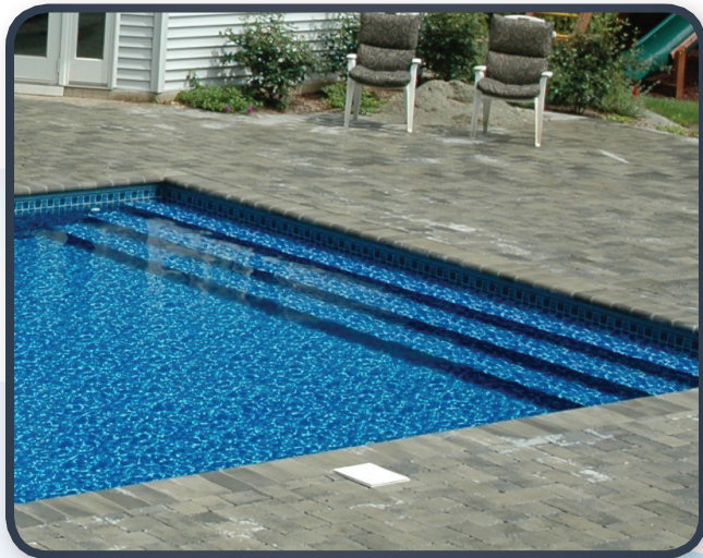
Full End Stair
